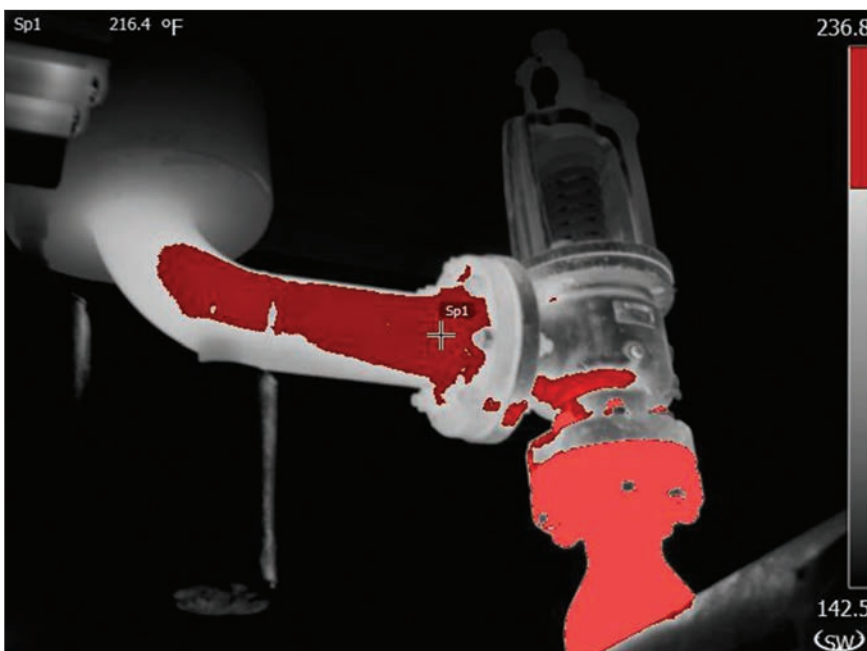
Fig. 9 - SV Leak detection
